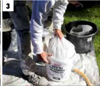
3 Tiltsett pulveret i spannet
