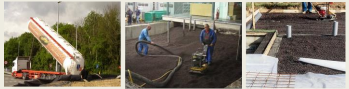
Figure 3: Blowing with vibrating plate levelling-compaction installation
