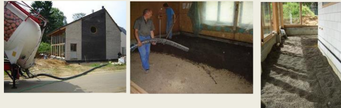
Figure 4: Blowing with manual levelling installation
