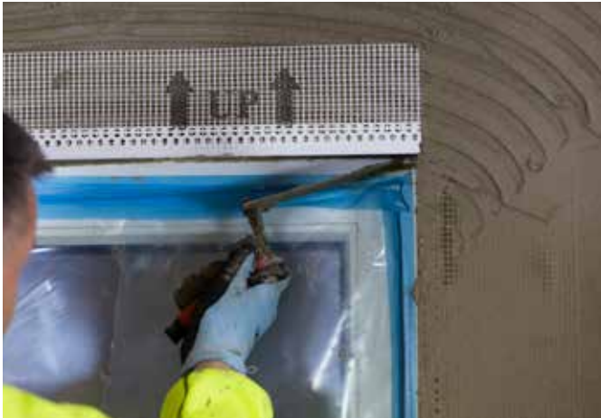
Over vindu monteres Mapetherm Driprnose Bead .
