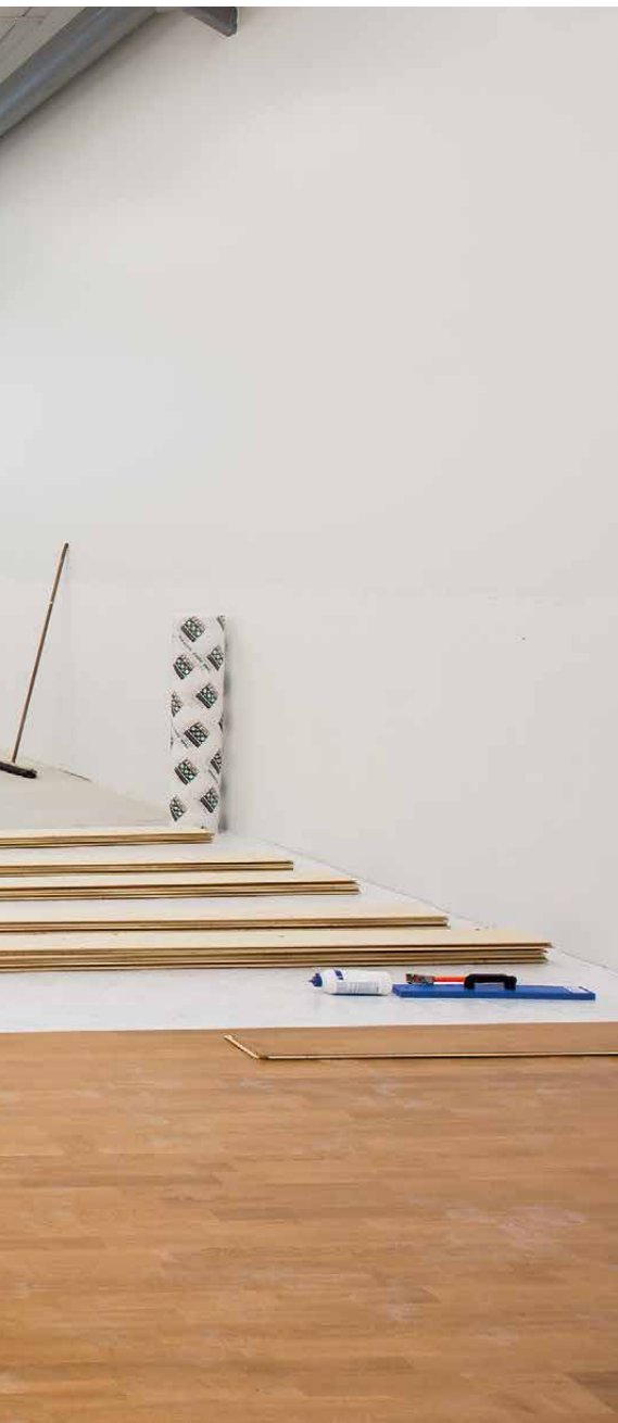
Figure 36. Spruce plywood installed directly on top of an existing floor
