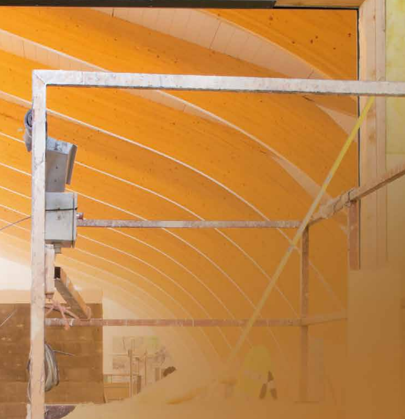
Plywood panel as a fixing base
