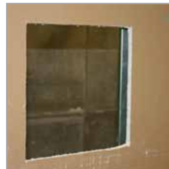
4 Hull klargjort for montering.
